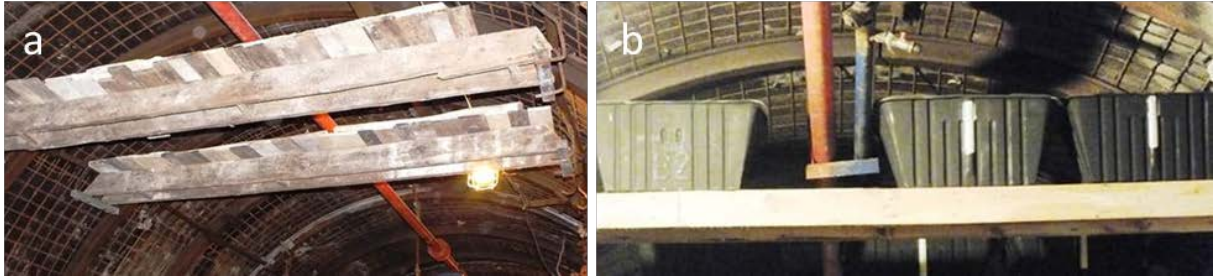
Fig. 2. Stone dust (a) and water (b) barriers in a mine working
